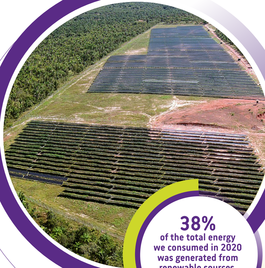
Timon Solar Power Plant
